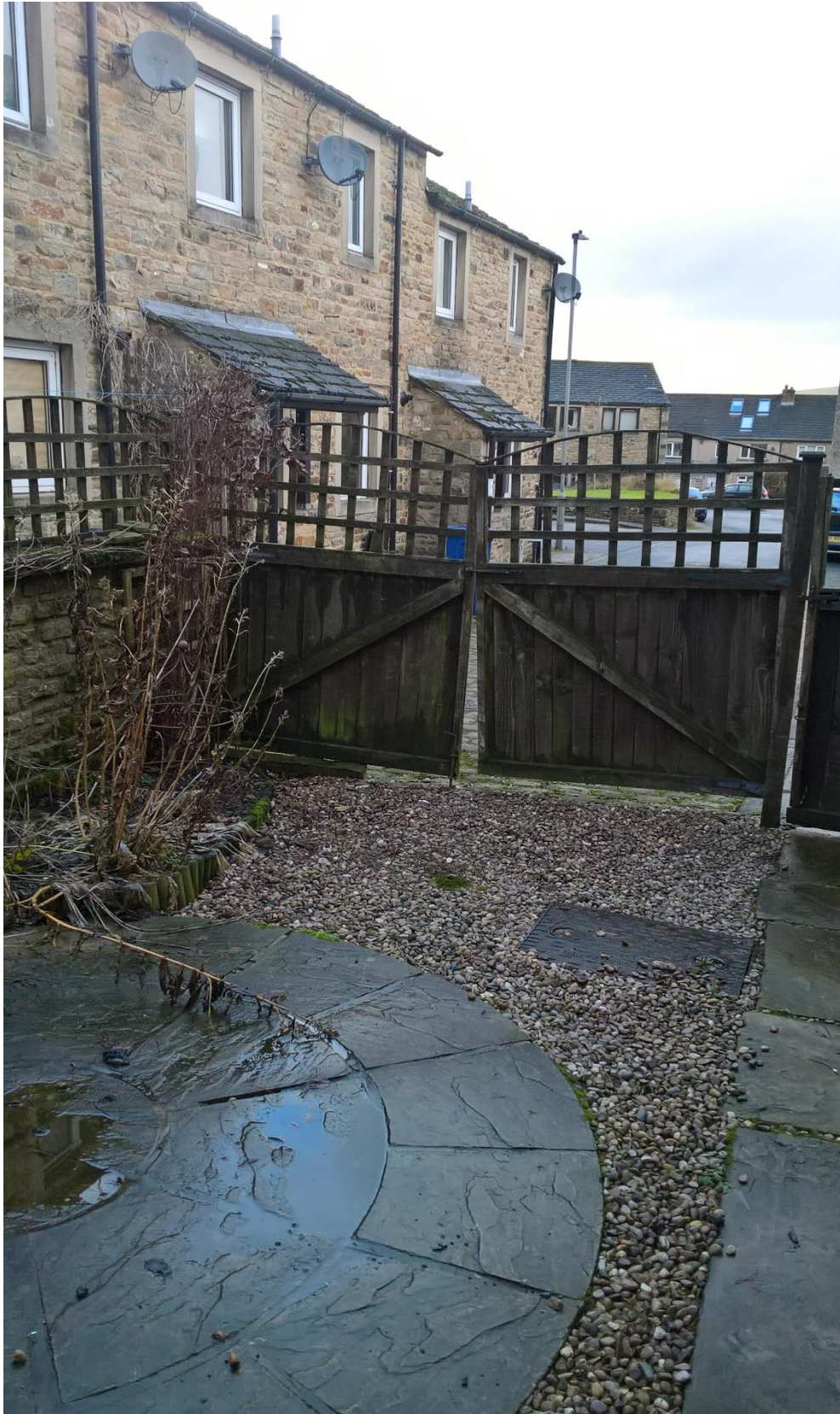
3. Exit of existing footpath on to Gordon Terrace from the back garden of No 124 Main St.
