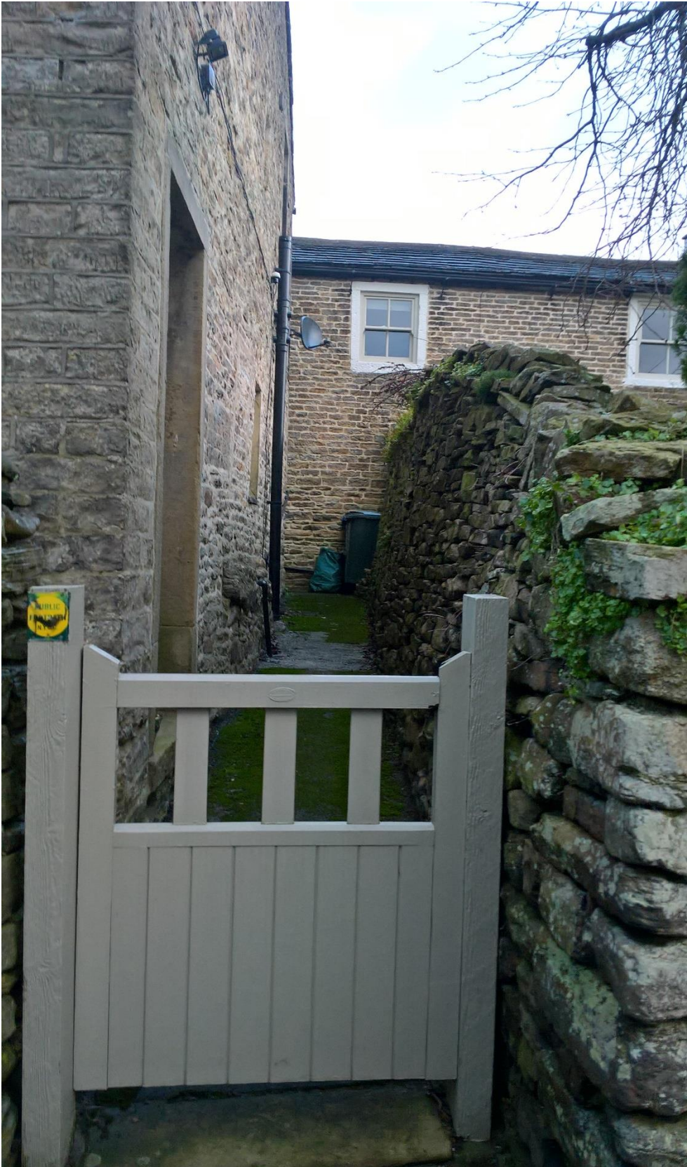
2. Hand gate at Point A on existing footpath.
