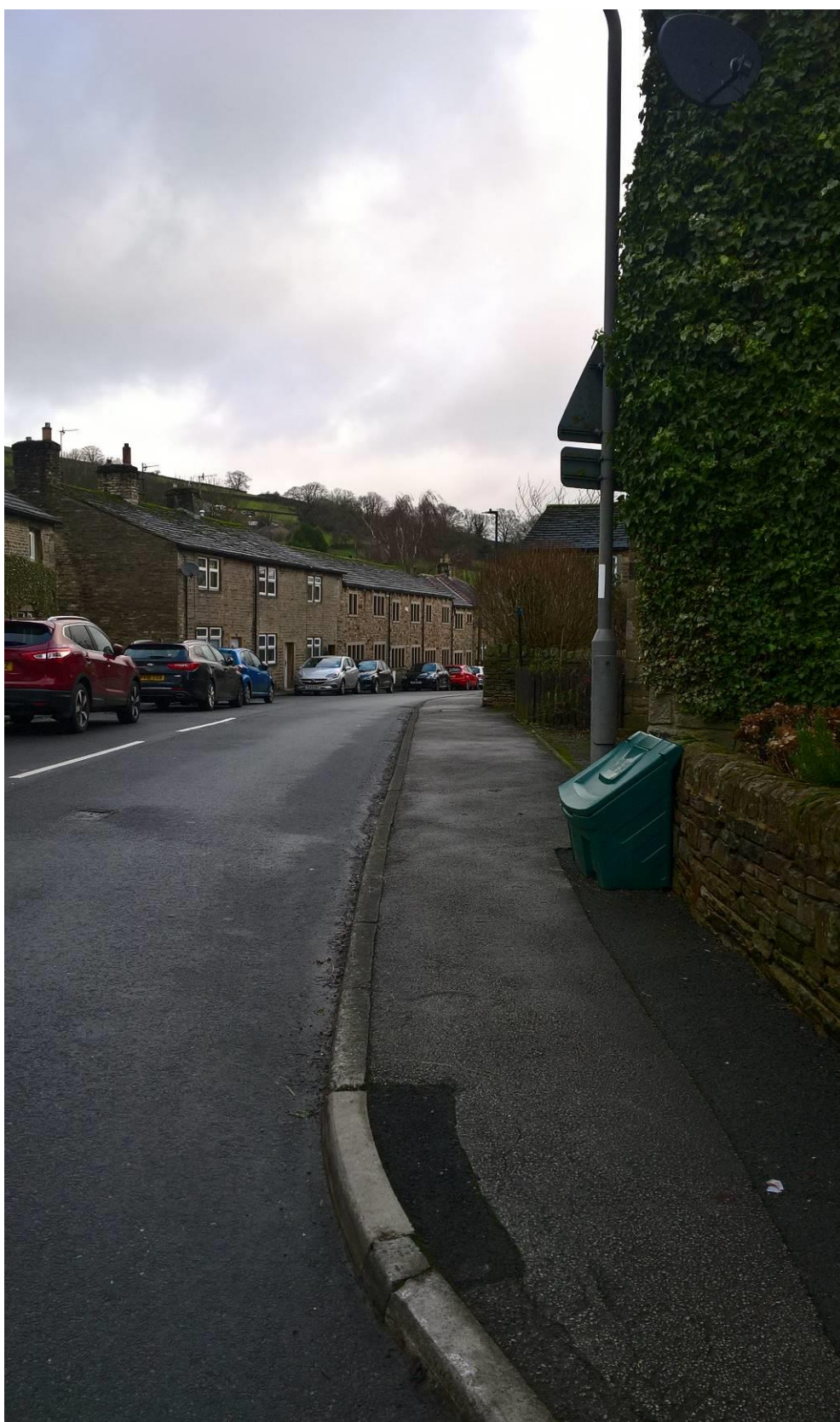
8. The end of the short section of roadside footway south of Point D.
